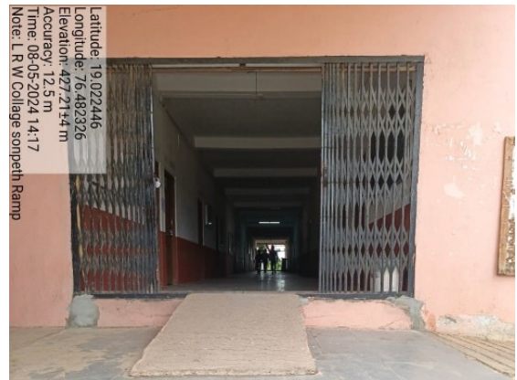
Ramp-Entrance to Library
